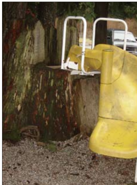
The deteriorating slide (above) in the Cedar Grove community playground is over 15 years old and isn’t accessible for children or parents who have physical disabilities.
